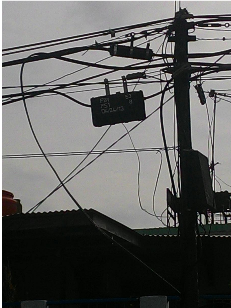
Gambar 10 Optical Distribution Point (ODP)
